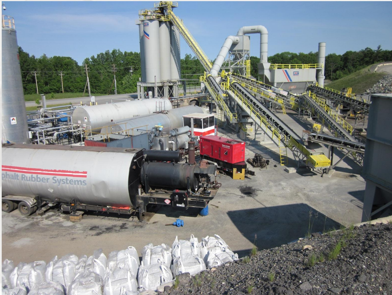
AR Blender Integrated with HMA Plant
